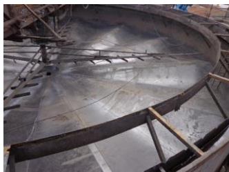
Thickener tank refurbishment at MMG Golden Grove
