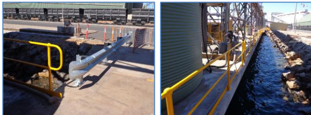
Installed handrailing/barricading at the Geraldton Port
